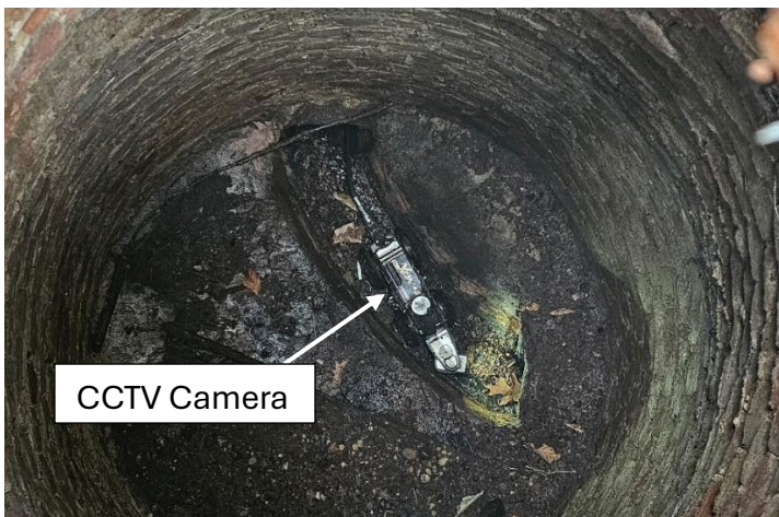
Inside View of Unlined Manhole and Sanitary Sewer Main
