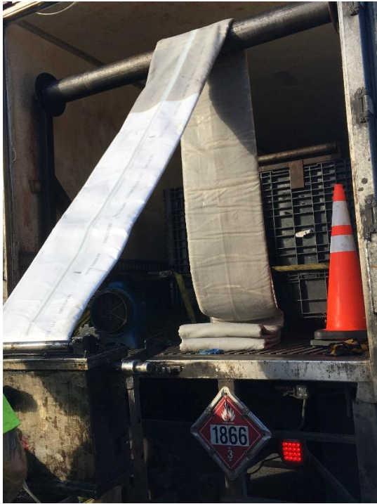
Installation of CIPP Liner
