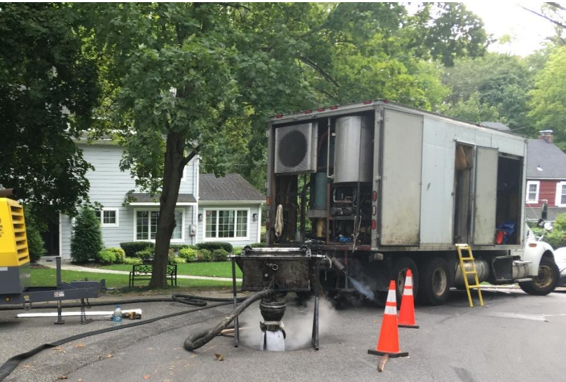
Steam Curing of CIPP Liner
